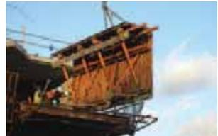
Figure 4 Steel shutter being removed from tunnelform after casting a bay
