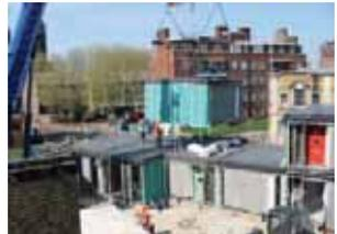
Flats being constructed with volumetric units – all the units shown were placed in one day
