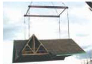
Pre-assembled roof structure being lifted into place
