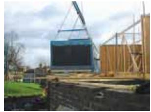
Volumetric unit being placed alongside panels
