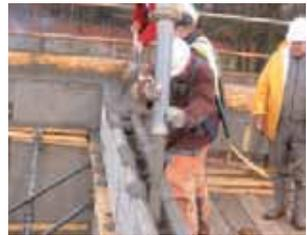
Concrete being poured into insulating formwork
