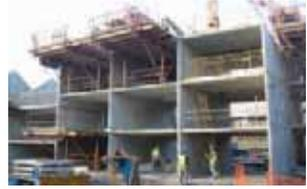
Figure 2 Tunnelform construction
