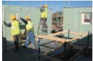
Closed timber frame panels being placed
