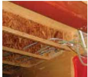
I beam timber joists
