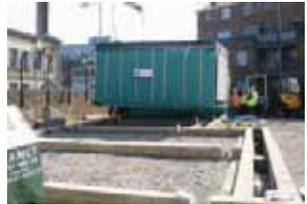
Volumetric unit being placed on levelled substructure
